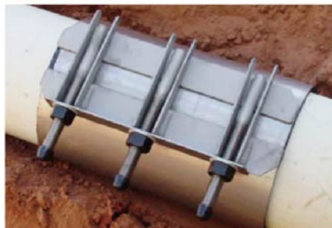
Step4 Use a tension wrench to sequentially tighten the studs to the recommended tension specified on the clamp.
