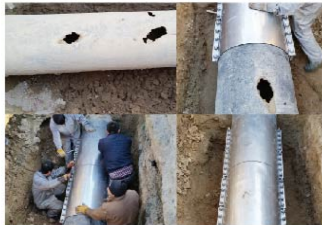
6. Zhuhong Lengthen Type Repair Clamp is used for fast repairing of long leakage of DN900 ductile iron pipeline of Jinan Water Group.
