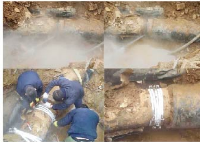
For the leakage of 20° degree elbow of DN450 heating pipe, Zhuhong Elbow Repair Clamps overcome this technical difficulty just in 10 minutes.
