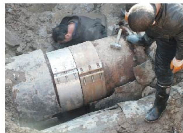
Shanxi Thermo-Power Corporation uses our DN500 Repair Clamp for their emergency repair of heating pipeline.
