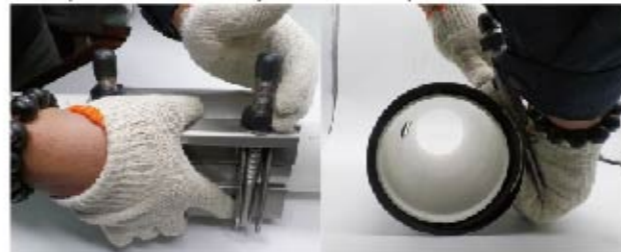
Step3 Assemble the clamp around the pipe by bringing the lock plate over the alignment lugs and hand tightening the nuts to hold it in place.
